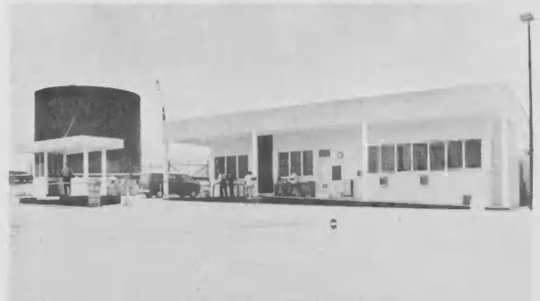
The new Industrial Services Building at Gate 2 since August 14 is the permanent headquarters for Lago's security personnel.
